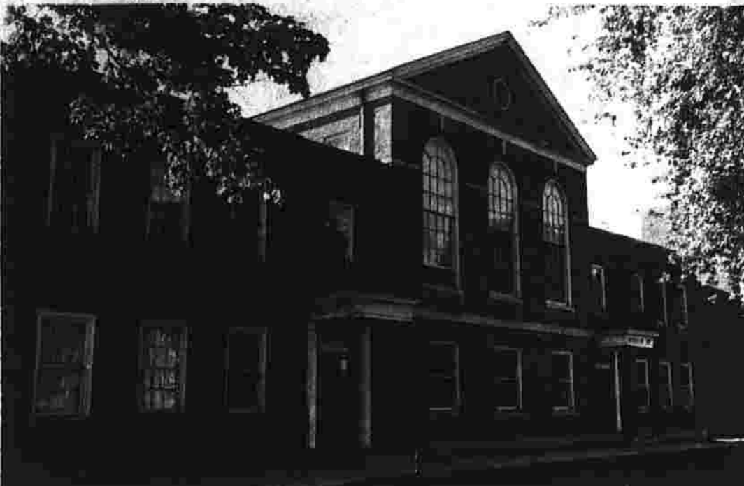
The West Side Recreation building on Cedar St., better known as the West Side Rec, is being razed this week to make way for a modern facility to be shared with the adjacent Washington School. The Rec has been the center of activity for several generations of West Side residents since 1921. (Herald photo by Pinto)
